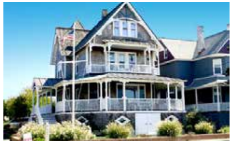
400 S. Bayview Avenue
